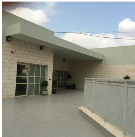
Mixed uses center kindergarten, day care and culture center Nes Ziona, architect Gaby Nussbaum
